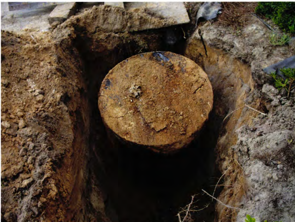
Picture 2: UST 531LaurelBB removal in progress.
